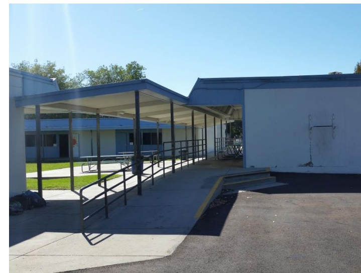
Photo -3 Some site improvement has been performed to improve accessibility.
