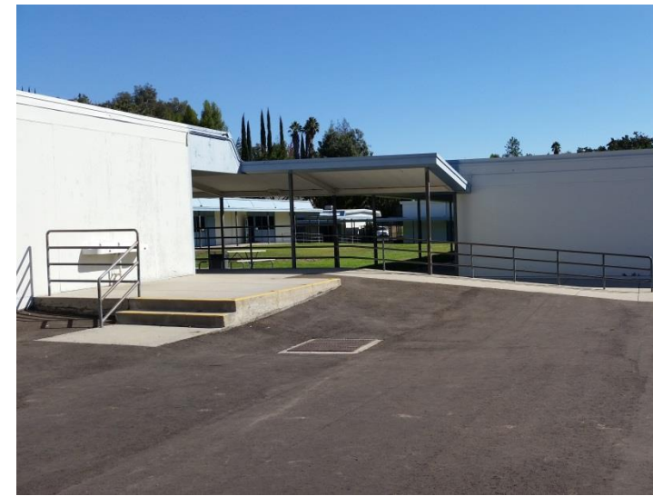
Photo -1 Stairs do not comply with accessibility standards.
